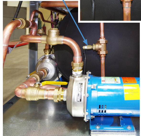
Auto Level Switch (this model shown is for Stainless Steel Tanks)
