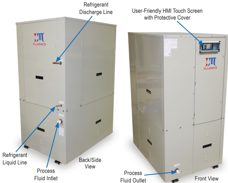
OC Refrigerant Connections: Discharge Line- 3/4", Liquid Line- 1/2"
