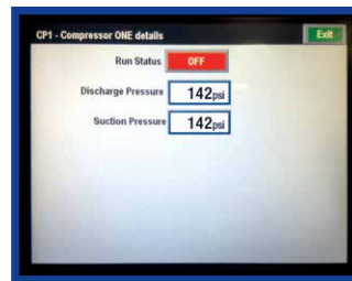
Compressor Operation Status and Pressures
