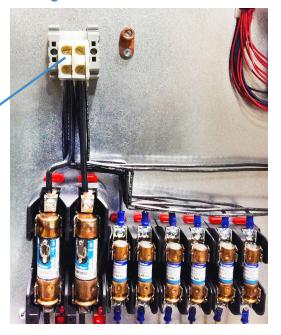
Some chiller manufacturers have multiple connection requirements before all power needs and functions are operational. All J&M Fluidics chillers come <u>standard</u> with **One Single Point Power Connection** for all functions and operations.
