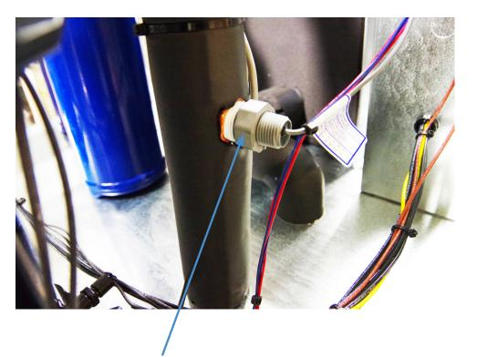
The water flow switch is a transmitter that senses the water flow of the chiller... If there is low flow or even no flow, the water flow switch will shut down the chiller for protection.
